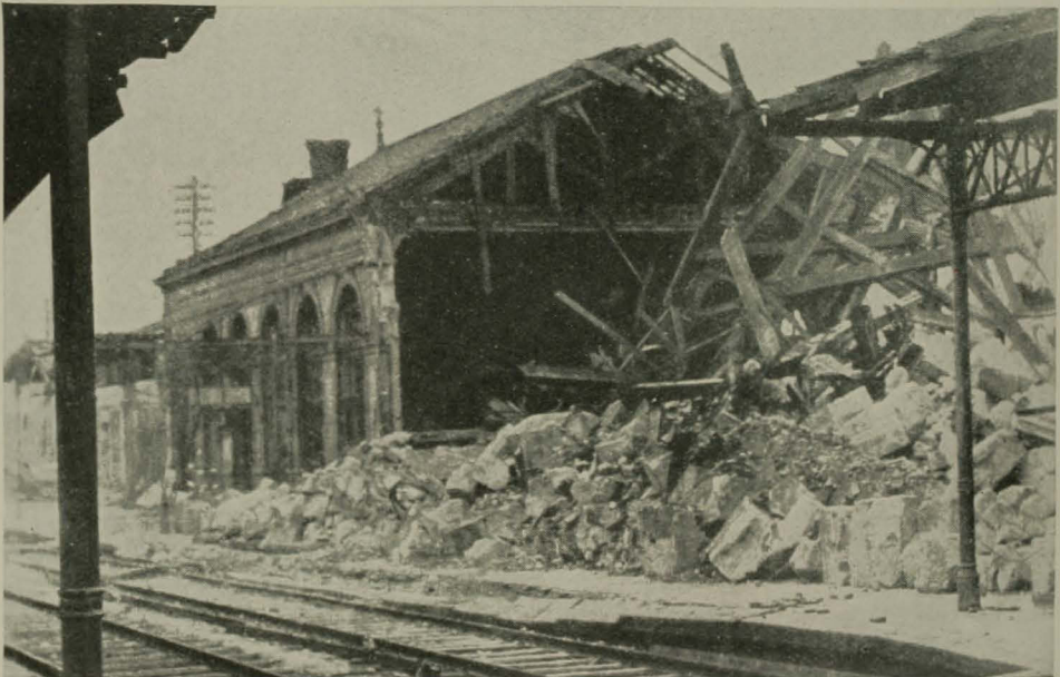
Railway Station at Sedan
