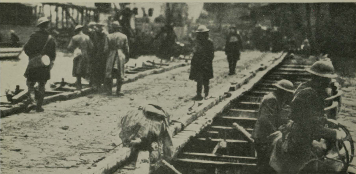
Ponton Bridge Constructed by 5th Division Engineers Near Dun-sur-Meuse
