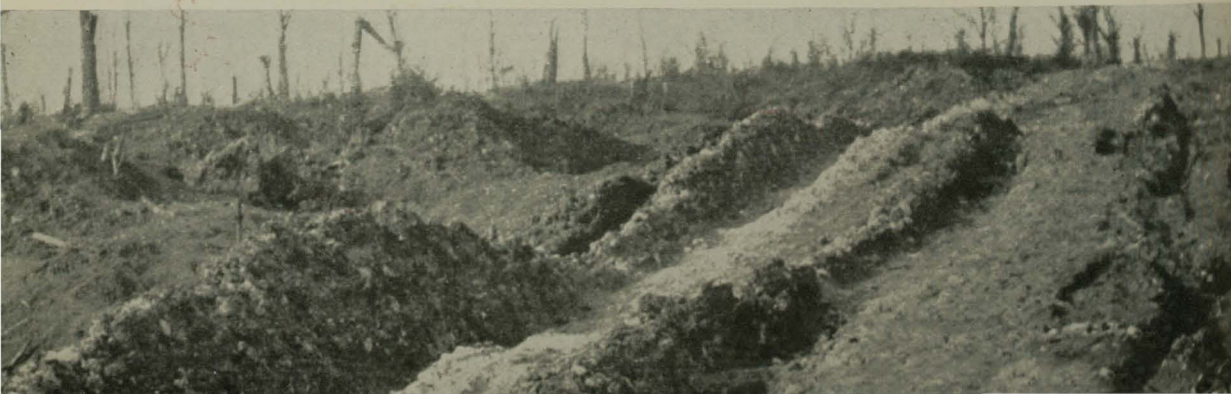
Results of Traffic on the Avocourt-Malancourt Road Built Over No Man's Land
