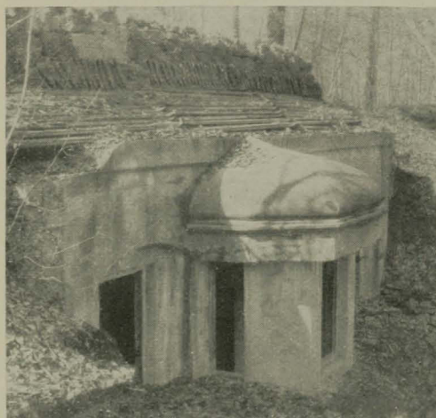
Concrete Dugout in Champ Mahaut
