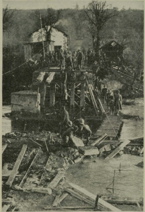
Engineers Building a Bridge Across the Meuse Near Pouilly After the Armistice
