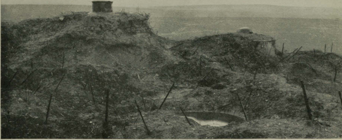
Steel Observation Turrets at Fort Douaumont
