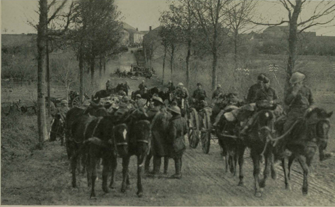
Troops West of Bar, Compelled to Pass Around Bridge Being Repaired, November 3, 1918
