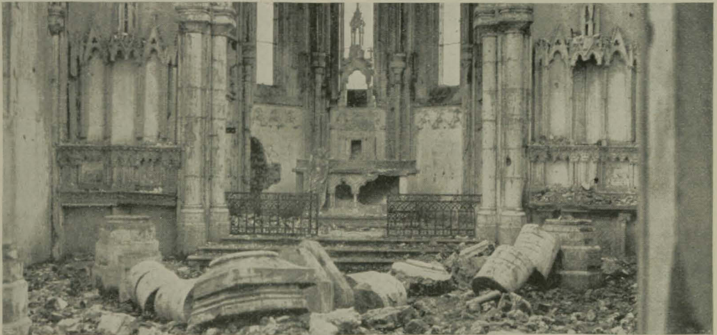
Interior of Beaumont Church
