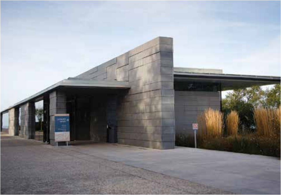
Exterior of the Visitor Center. (ABMC photo/Warrick Page)
