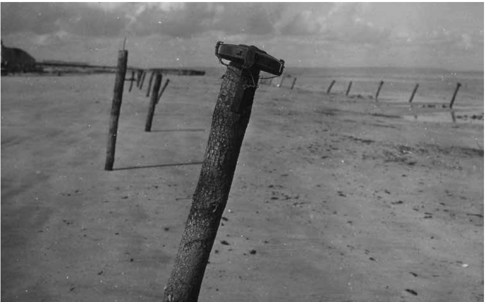
The German Army installed formidable defenses on the beaches of Normandy, including teller mines attached to stakes. (National Archives)
