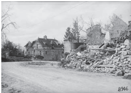
The town center of Belleau, just north of Belleau Wood, suffered heavy damage during the war.
