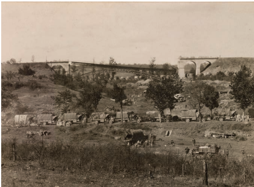
Damaged bridge at Flirey. Note traffic jam of trucks in the foreground.
