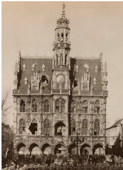
The damaged Oudenaarde city hall, 1918.
