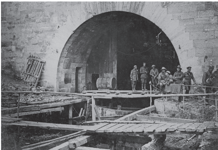
Close-up of the Riqueval Tunnel mouth.
