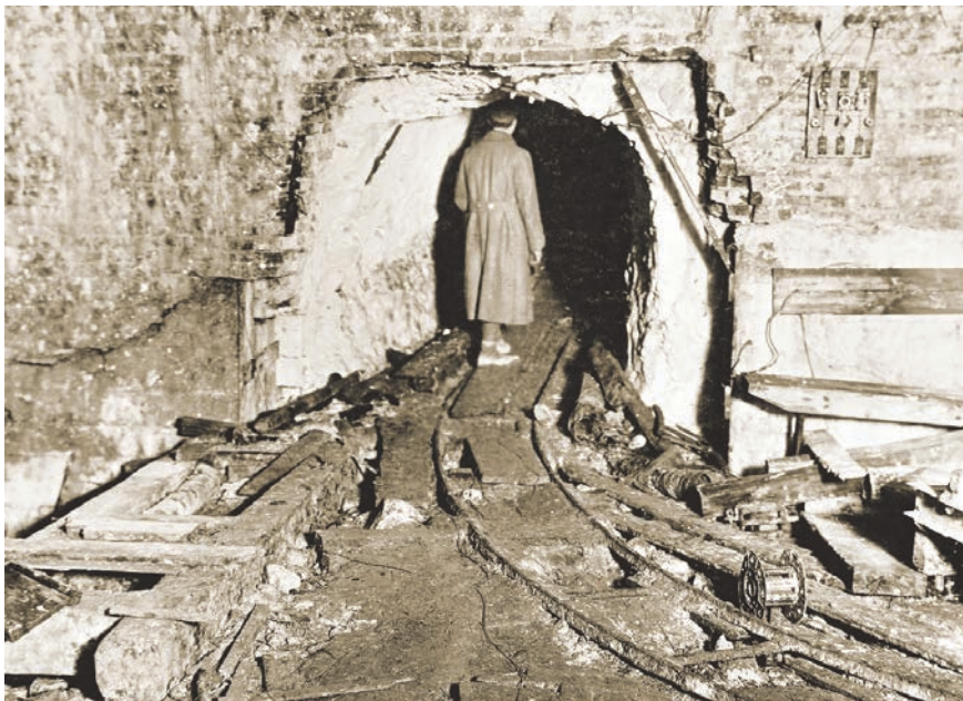
The Germans honeycombed the ground around the tunnel with shelters equipped with lights and small tram rails.
