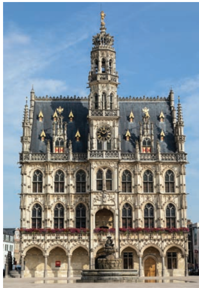
The repaired city hall in 2018.
