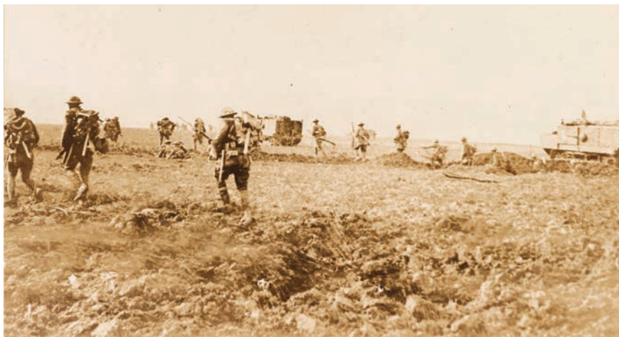
American troops advance on Cantigny with French tanks.
