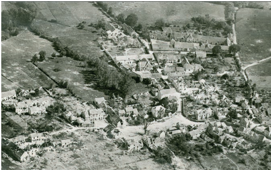
The shell-scarred town of Bouresches just south of Belleau Wood after the fighting in 1918.
