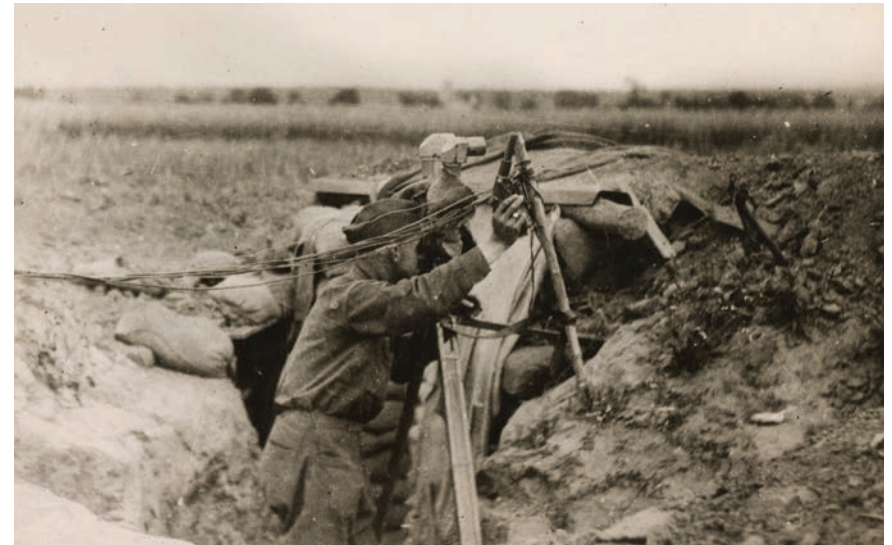
An artillery observer with a tripod periscope and telephone lines to his artillery battery. The observer was essential to accurate artillery fire.
