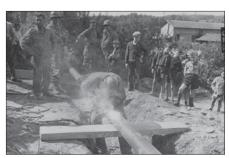
Engineers weld a gasoline pipeline into place to meet the demand for fuel by the advancing Allied forces.
