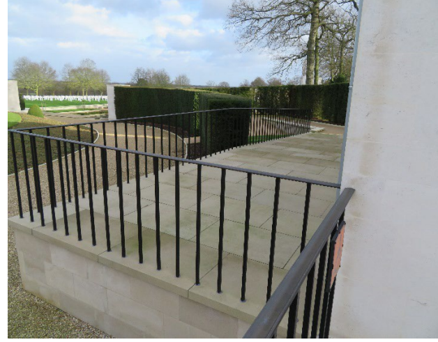
Ramp from entrance courtyard to lower level.
