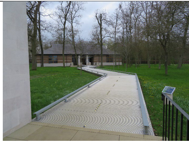
Raised walkway to Visitor Center.
