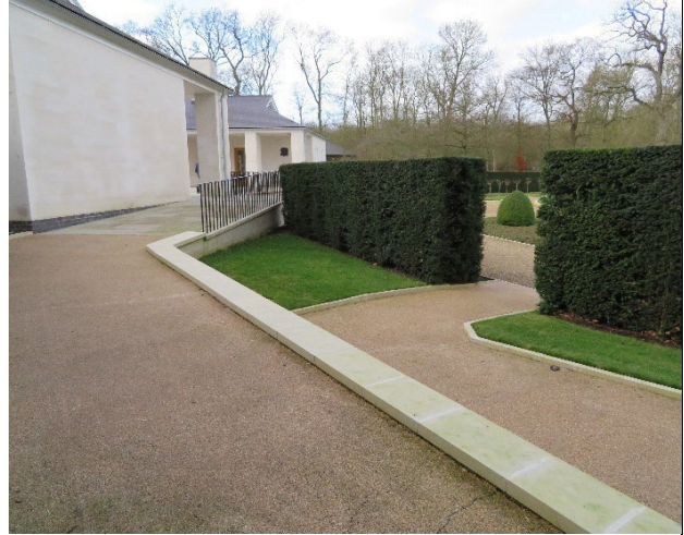
Ramp from main courtyard to flagpole area.
