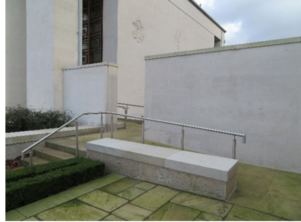
Ramp from Wall of the Missing to Memorial Building.
