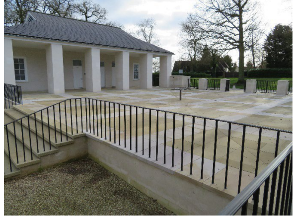
Level entrance courtyard and accessible toilet.
