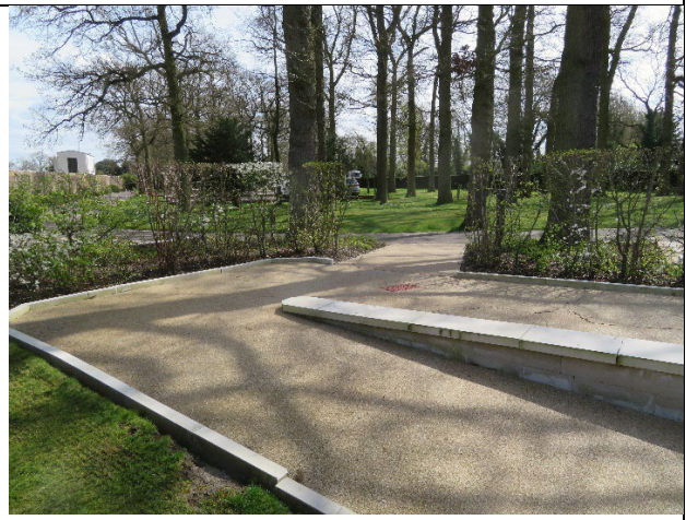
Exit from ramp to car park.
